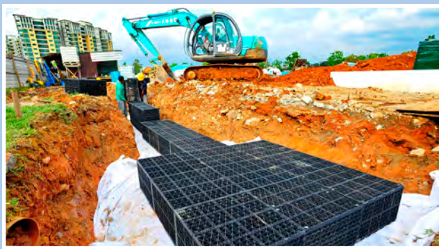
VersiTank® Infiltration System installed at a park
